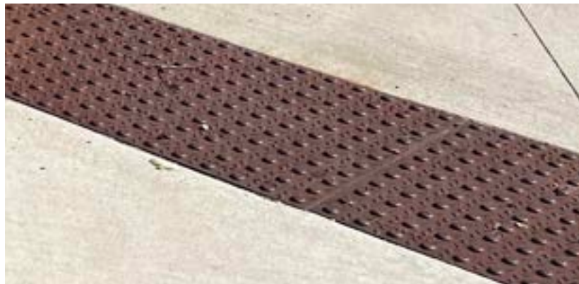
Cast Iron Detectable Warning Surface
