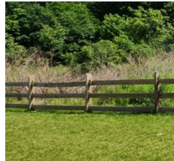
Existing Post & Rail Fence (to be relocated)
