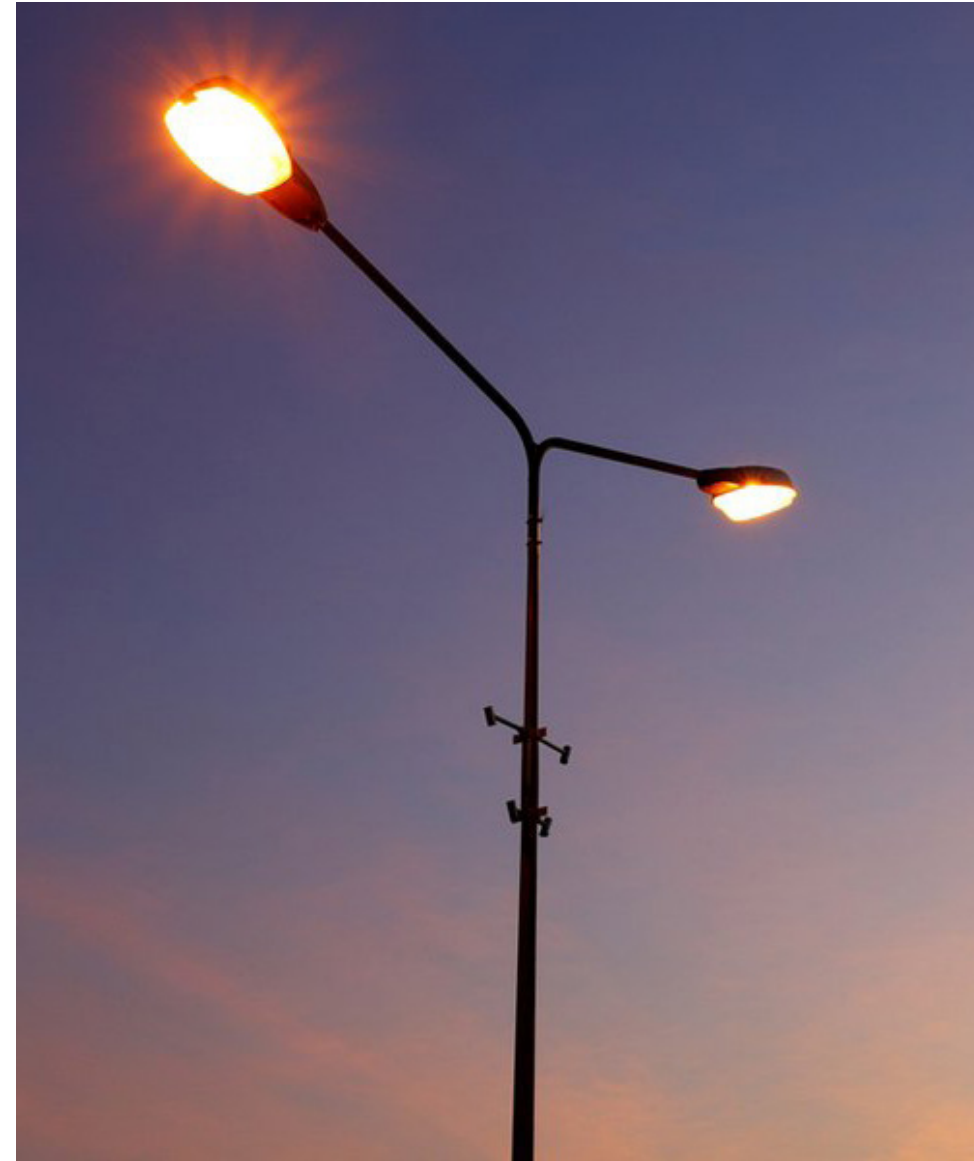
Philadelphia Streets Department Street Light Pole
