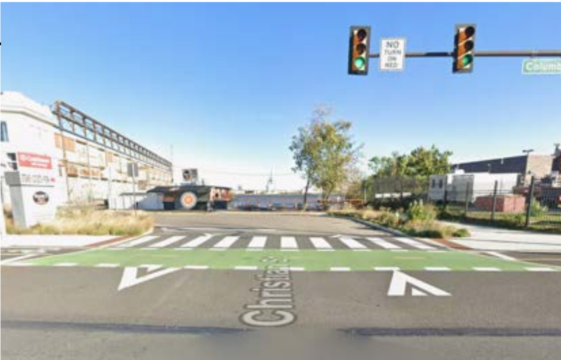
Raised Pedestrian Crosswalk
