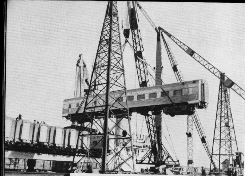
Passenger cars, destined for South American use, are picked up by the 100-ton derrick and deposited on the ship's deck. This is the largest privately owned water-side derrick on the East Coast.
