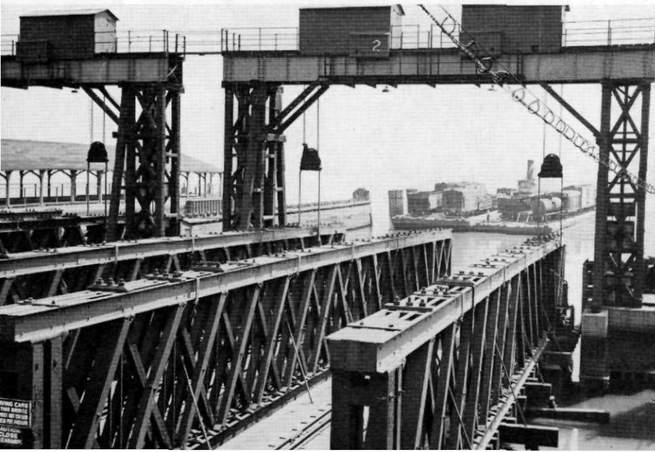
Two car floats move into the float bridges (Pier J), from which point cars will be moved to yards for further handling.
