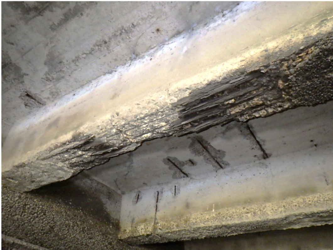
Photo 6: Severe deterioration of the bottom of the concrete beam.
