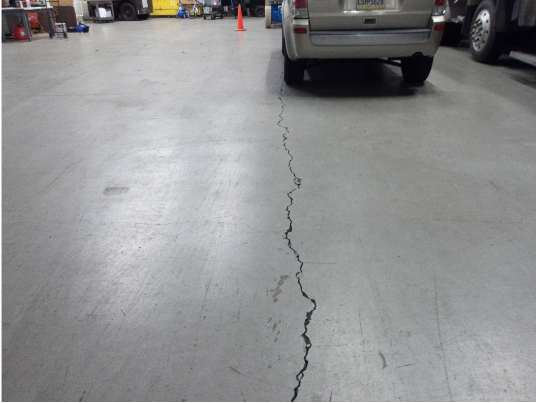
Photo 3: Wide crack in the interior of the building.
