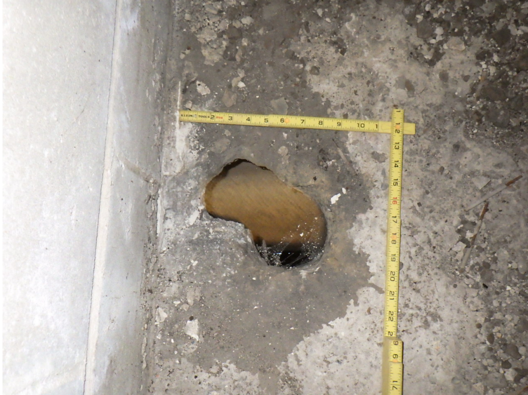
Photo 7: Full depth hole in the concrete deck.
