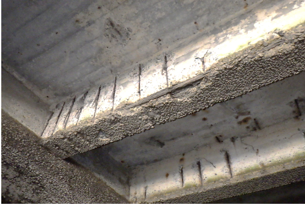
Photo 5: Reinforced concrete beam with exposed reinforcement.
