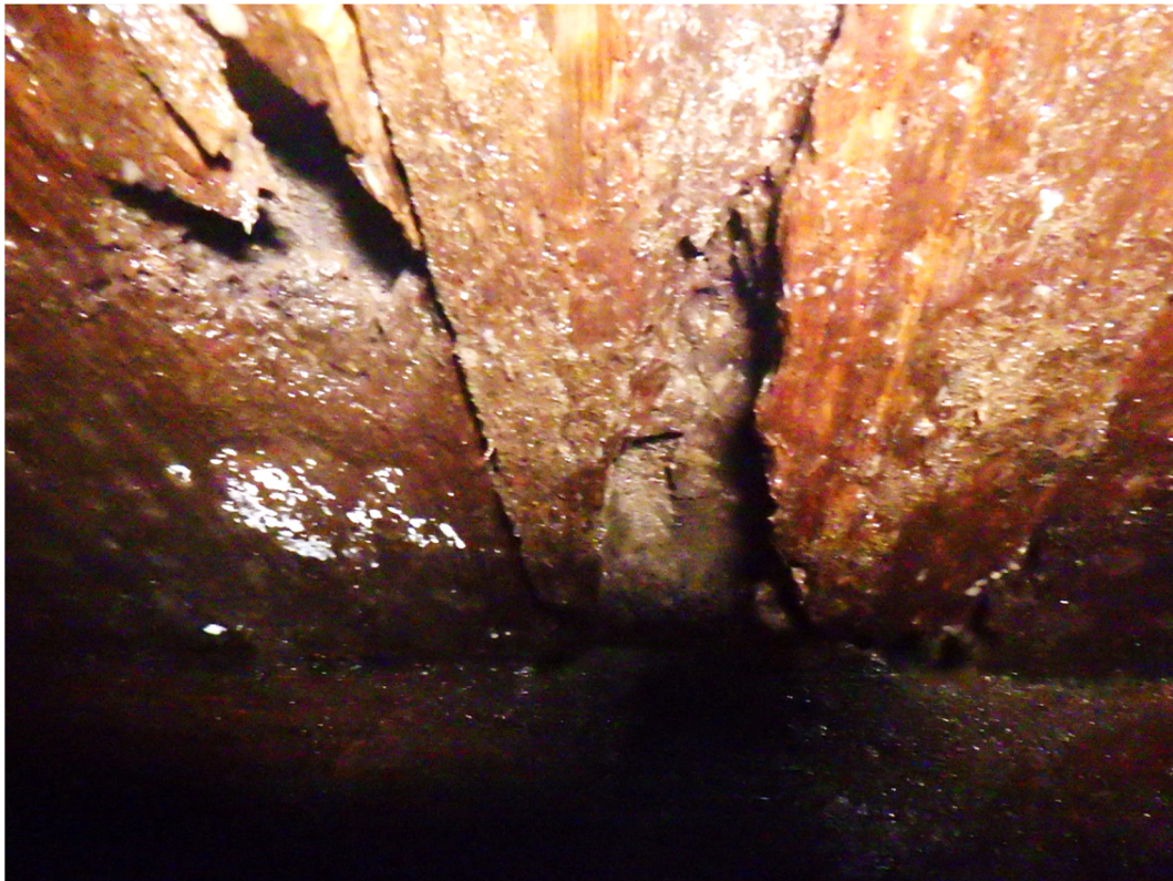
Photo 4: Broken timber decking.
