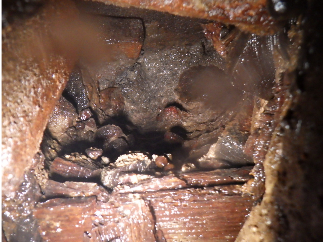
Photo 5: Missing timber deck members with exposed fill material.
