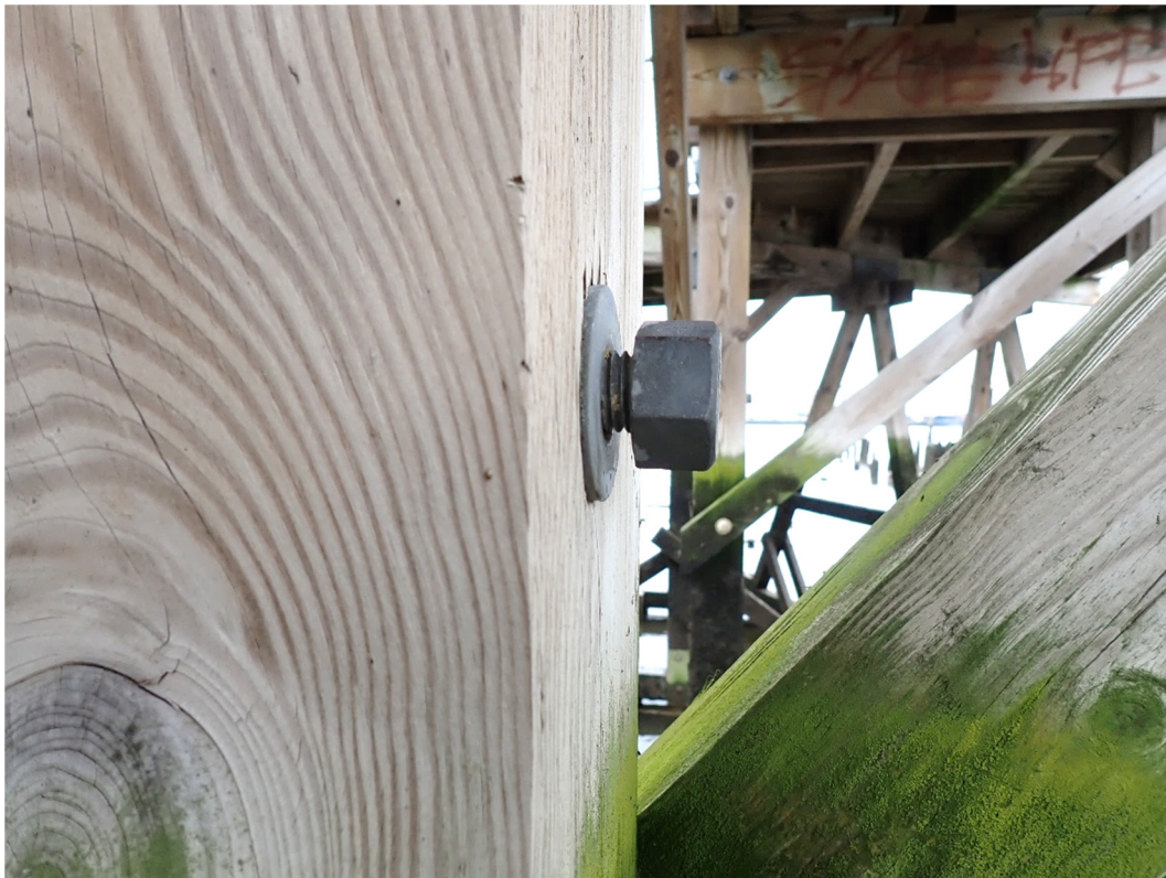
Photo 2: Typical loose hardware found throughout the structure.
