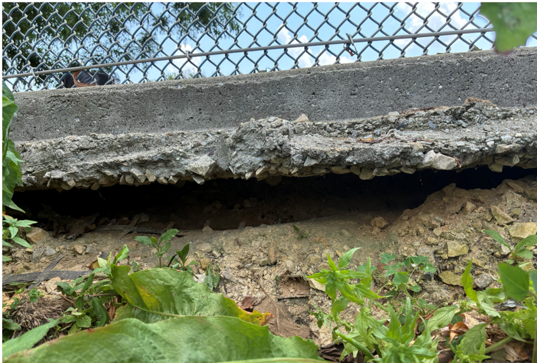
Photo 4: Interior of pier looking at the missing Grosoxx and void below the concrete.
