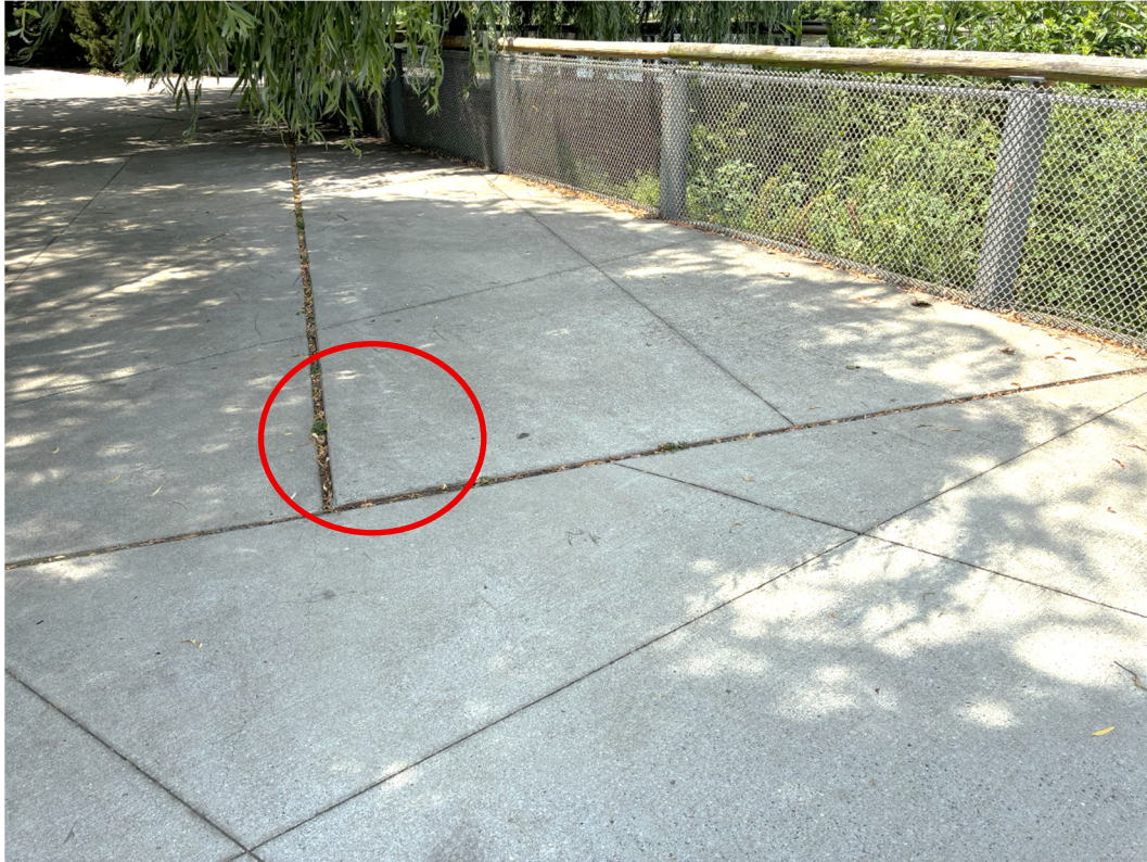
Photo 5: Uplifted concrete sidewalk on top of the pier.
