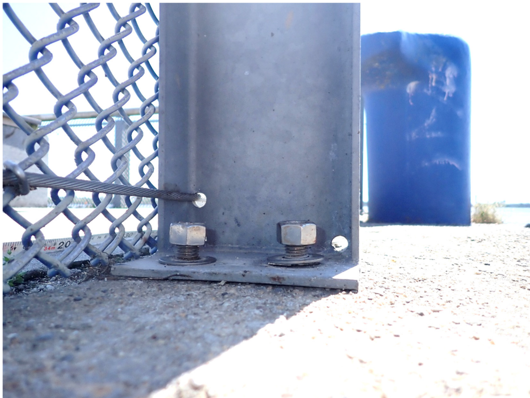
Photo 2: Loose fence post anchor bolts.
