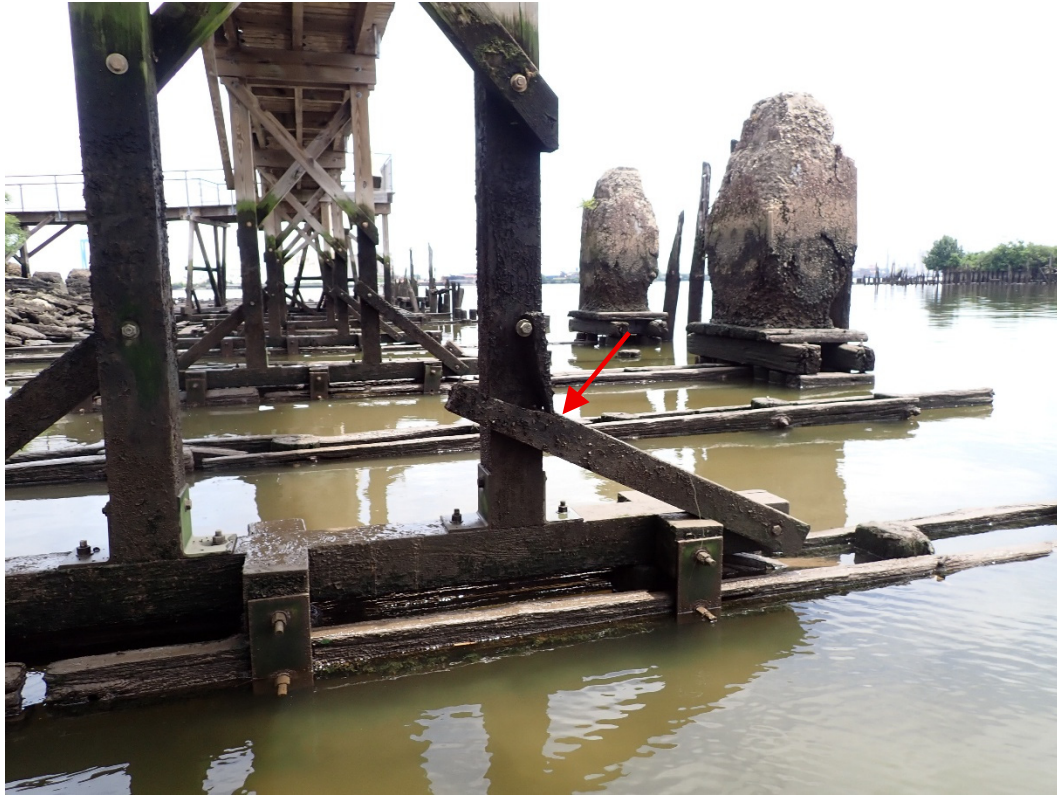
Photo 3: Damaged cross bracing at Bent 5 to be replaced.
